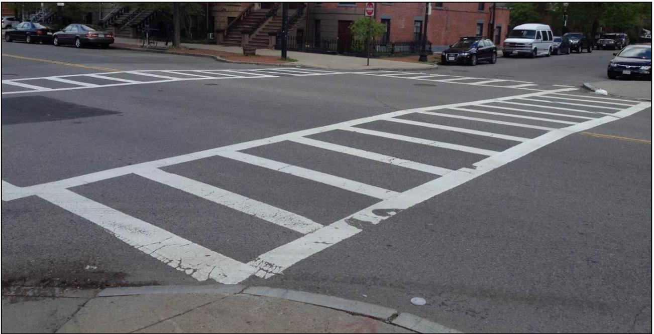
**Figure 7:** Possible crosswalk marking ("ladder")
