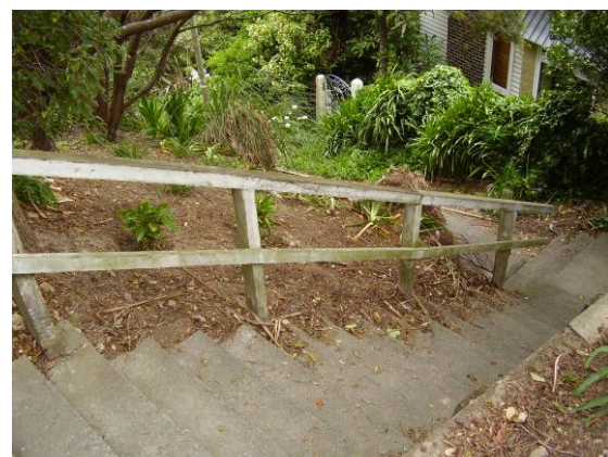
Handrail and walkway looking scruffy
