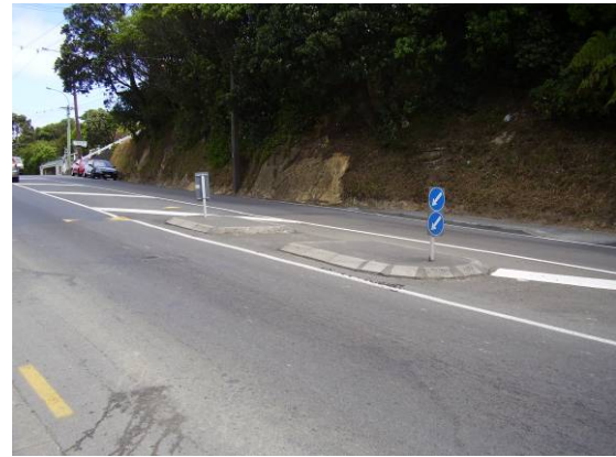
The alternative route without footpath
