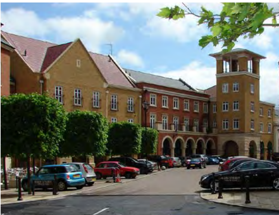
above: Concourse area within the Waterside development
