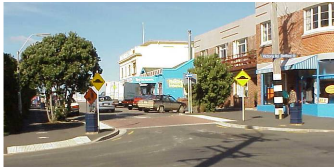
Figure 4: Example of a pedestrian platform installed at an intersection
