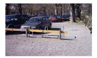
Figure 29: Wrongly installed bike stand
