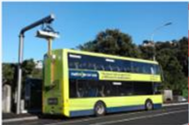
Battery electric bus charging infrastructure
