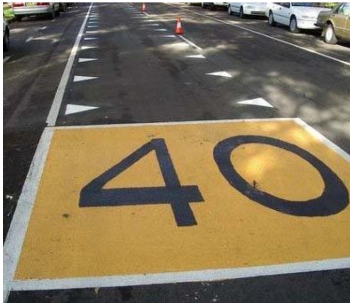
Figure 7. Painted school thresholds and dragon's teeth markings used at all 40 km/hr school zones in NSW
