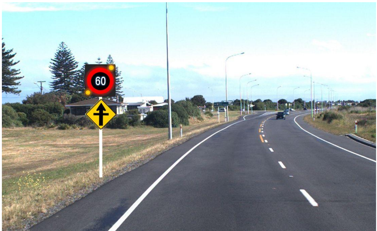
Figure 12. Example Rural Intersection Active Warning System (RIAWS) sign, so far used for focus group purposes, which in principle may be applicable to rural schools at intersections, to mitigate the risk of serious harm side impact collisions.
