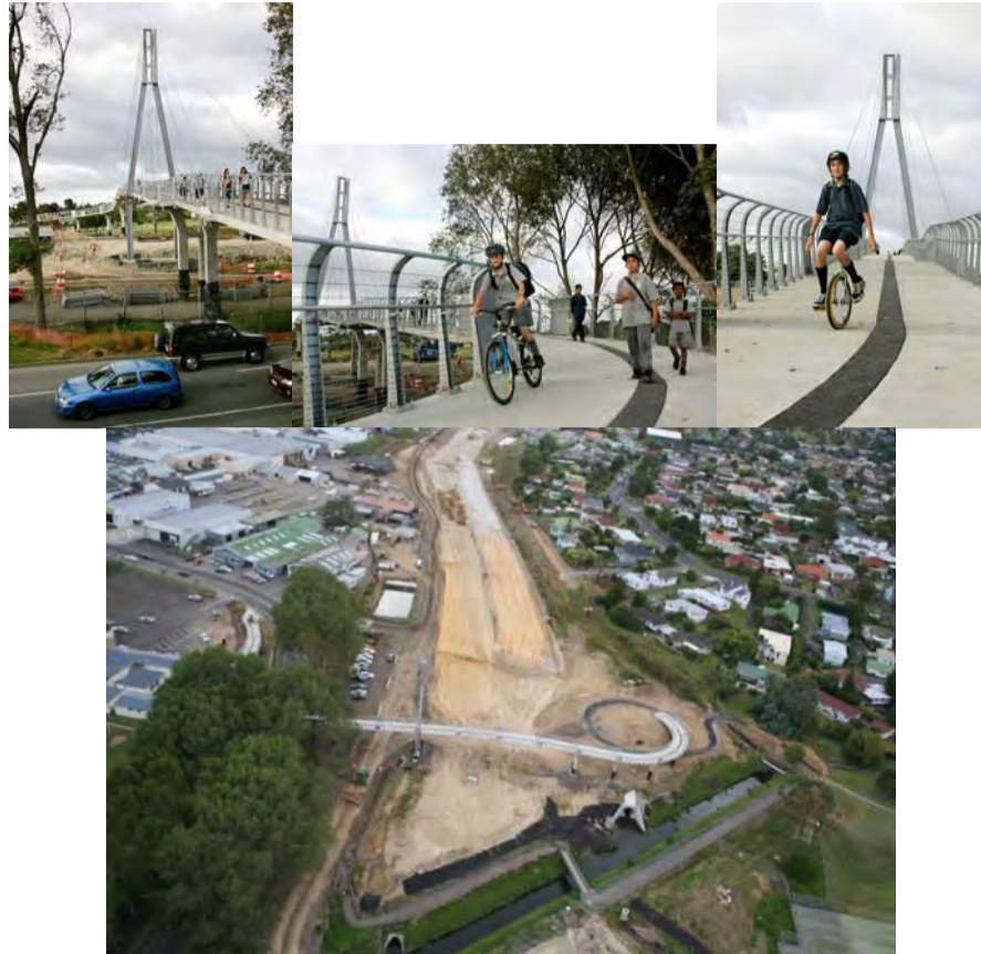
Figure 4, Images of the Keith Hay Bridge, Mt Roskill Extension under construction
