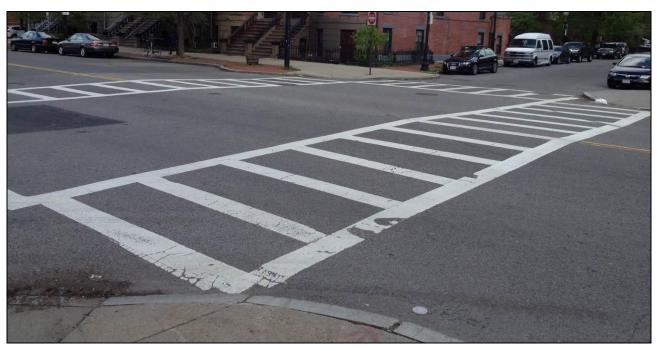
Figure 7: Possible crosswalk marking ("ladder")
