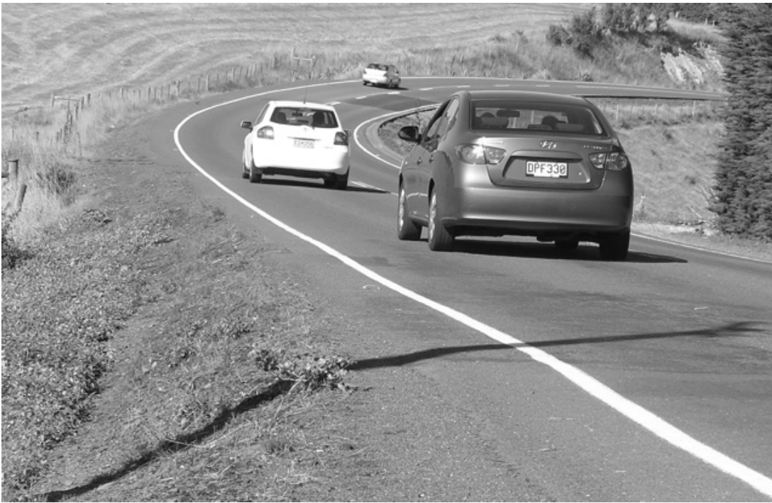
Figure 4. A closer view of the corner they were walking, showing narrow verge, uneven surface and steep unstable slope.
