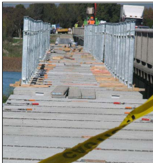
Clip-on bridge under construction for cyclists and pedestrians, Napier
