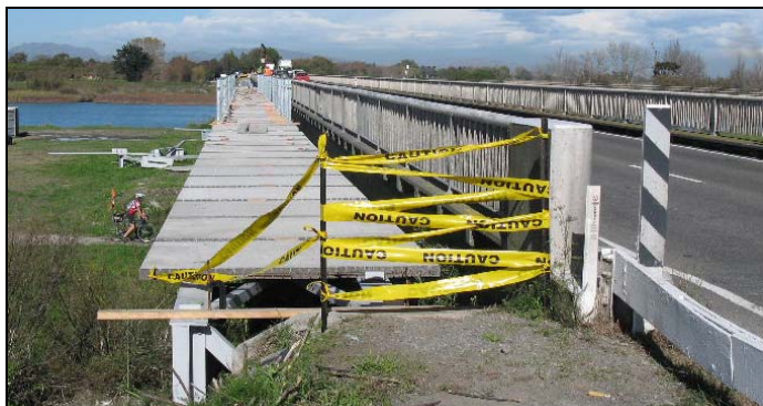
Clip-on bridge under construction for cyclists and pedestrians, Napier
