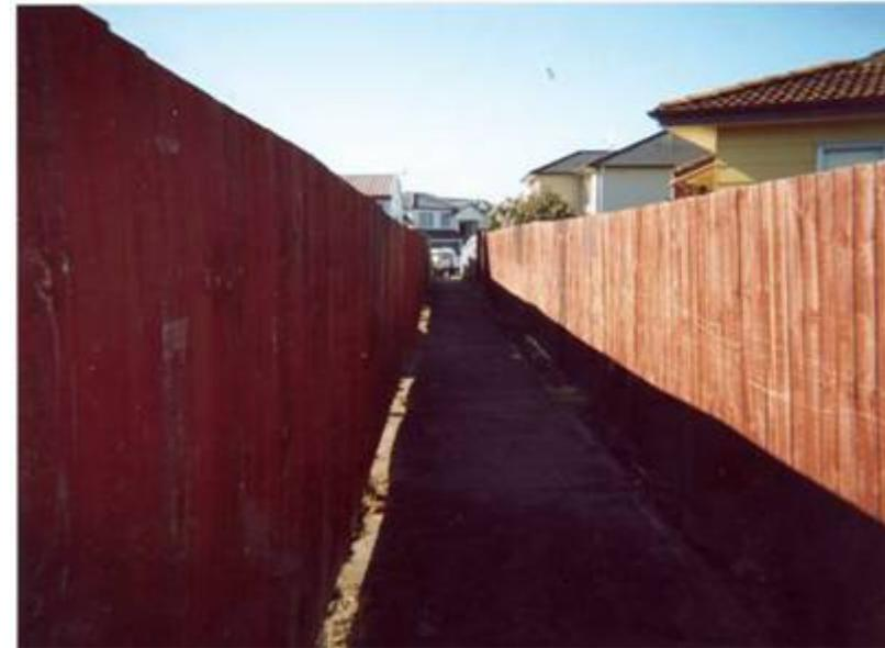
**Dislike: Convenient but water collects in heavy rain to 6" deep and remains until dried by weather (Glenhaven to Piriti Walkway)**
